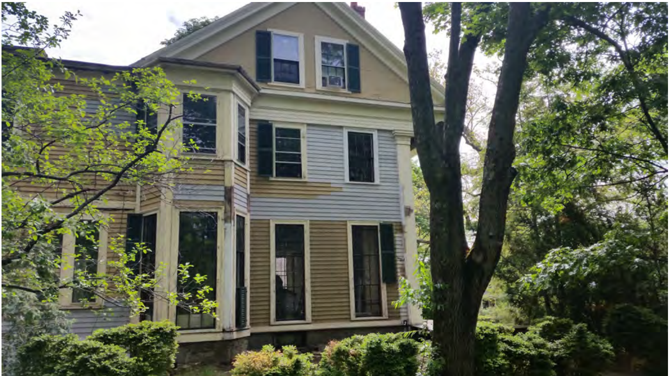
CPC Phase I work: Cherry St. façade work completed—porch demo, new window & siding
